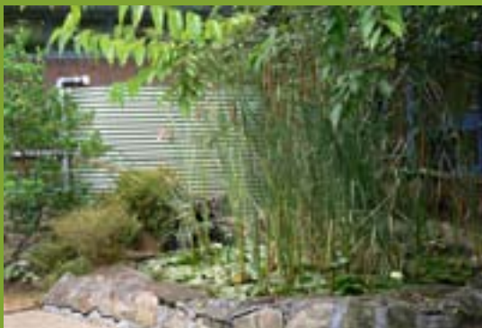
One of the many rainwater tanks used to mitigate storm water runoff and provide water for gardens, lawns and other maintenance tasks
